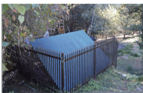
The filter tank is located on the slope of the mountain. The photo is with the lid open
